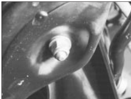
7.3 One of the nuts and bolts securing the lower arm to the subframe
