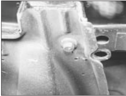
16.8 One of the rear suspension crossmember mounting bolts
